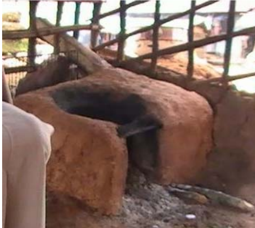
Figure 6. Energy saving cook stove before the kitchen wall is covered.
