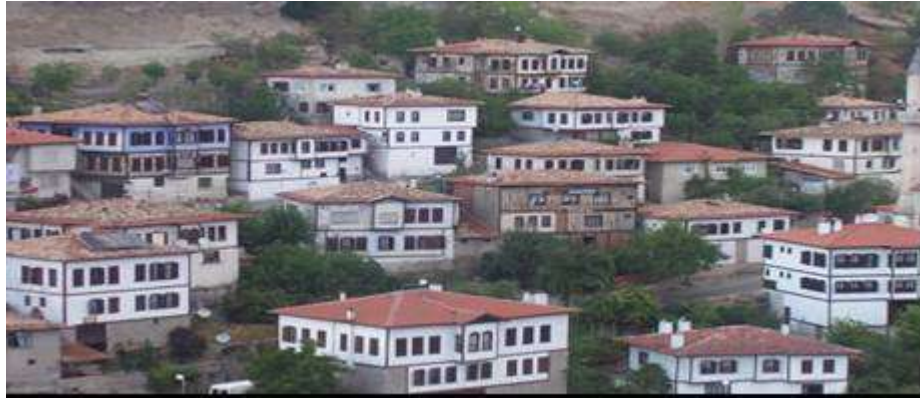
Figure 2. Architectural character of historical environment in Safranbolu.
