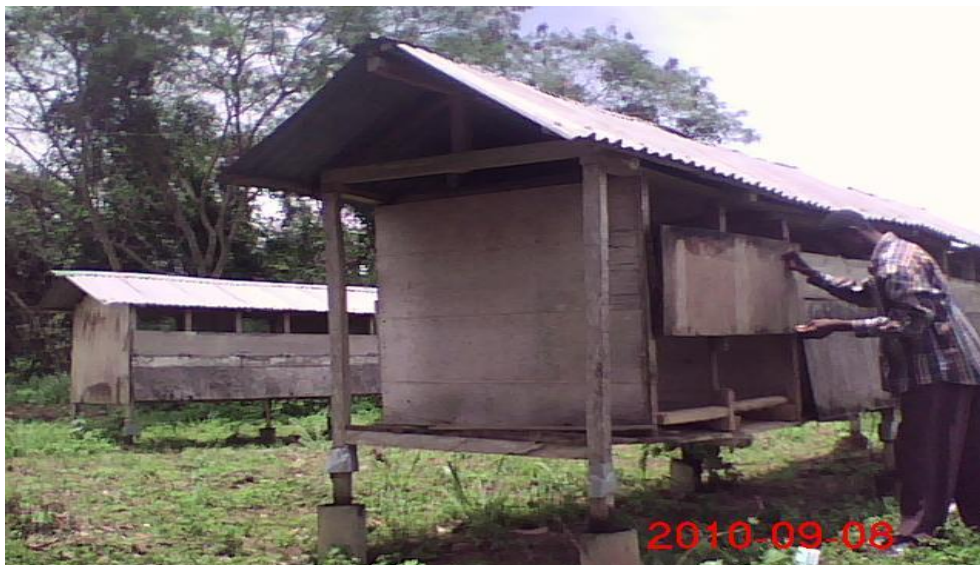
Figure 4. Two of the four experimental housing built with wood showing pens in the 45° (background) and 90° (foreground) orientations buildings.
