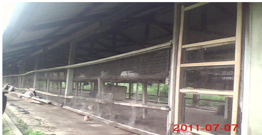
Figure 5. Experimental housing built with wood showing rabbits in their individual pens in 100% side opening building used as control, present conventional building.
