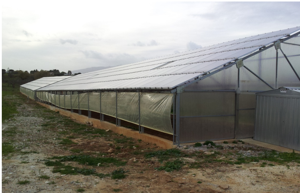
Figure 1. PV greenhouses of the case study.
