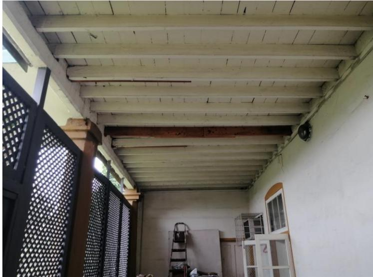
**Figure 3.** Show the suspended floorboards which have received repairs/restoration works in such a way that follows the existing construction method. This causes minimal disruptions to the character of the heritage building and was deliberately left unpainted to aid easy identification and appreciation of restorative efforts.
