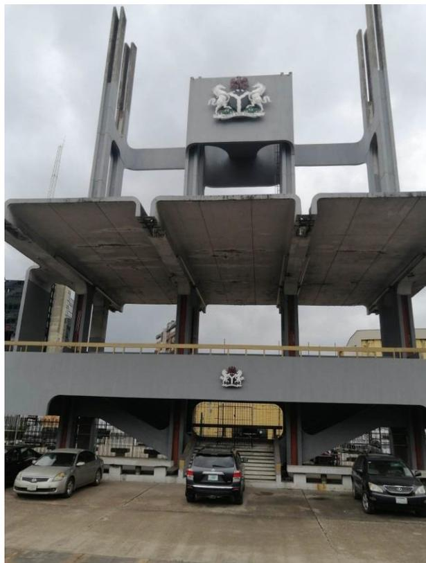
**Figure 4.** Picture showing portion of the independence entrance with the concrete roof cover in place, signs of wear and tear were noticed. The structure was recently painted.
