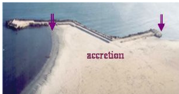
Photo 3. Local effects of accretion on the backshore - groin in southern part of Mamaia bay (13 I 2002).
