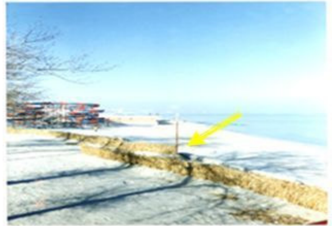
Photo 2. Soft beach protection measure with reed fences during cold season (13 I 2002).
