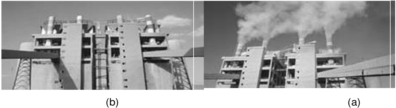
Figure 10. View of dust dispersion (a) before installing advanced hybrid filters (b) After installing advanced hybrid filters.
