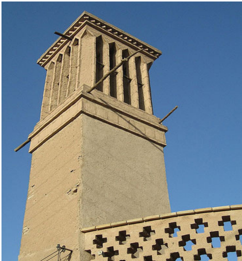
Figure 2. An instance of wind catchers in the warm and dry regions of Iran.
