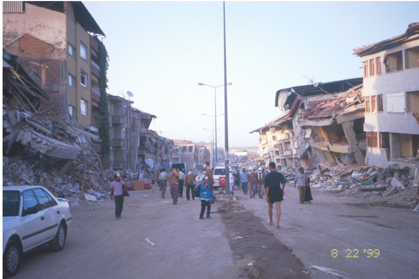
Figure 1. Marmara Earthquake and its devastation.
