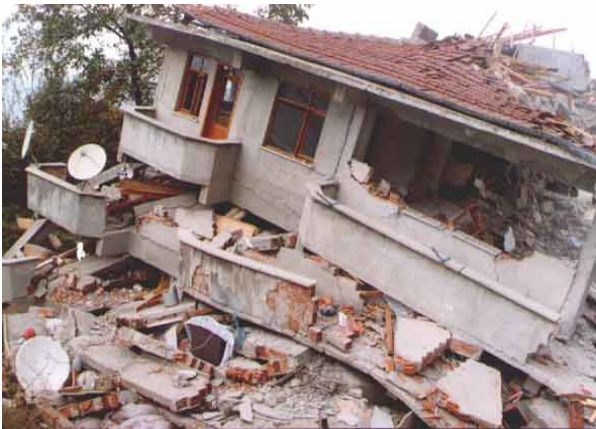
Figure 2. The URM building is very susceptible to seismic attack.
