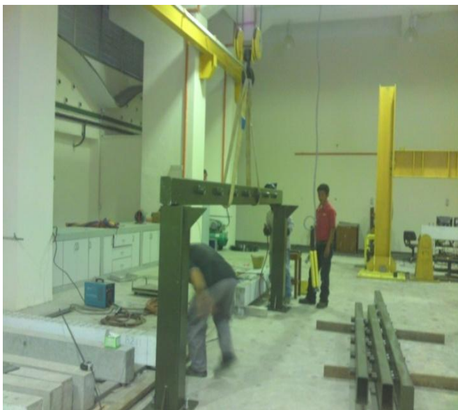
Figure 2. Construction of frame steel.
