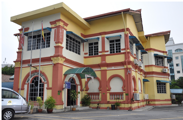
Figure 3. External facade of old building 2.
