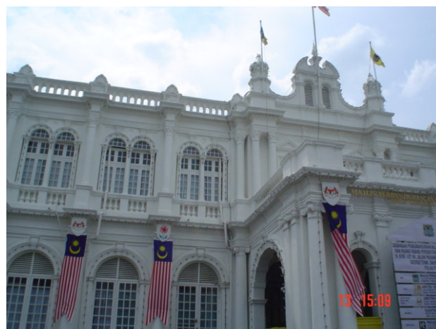
Figure 2. Exterior of old building 1.
