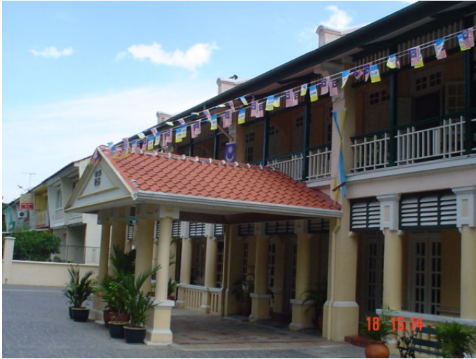
Figure 4. Exterior of old building 3.
