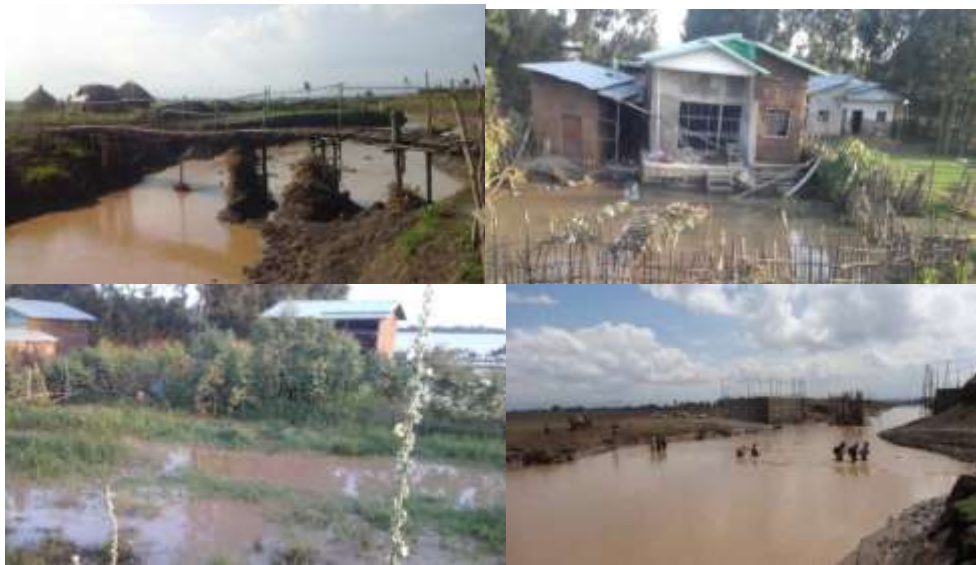
Figure 7. Flood impacts on properties and infrastructures.
