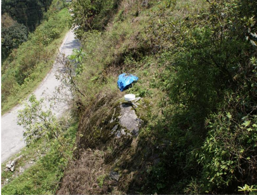
Figure 4. GPS Reference station in Bakthang slide.
