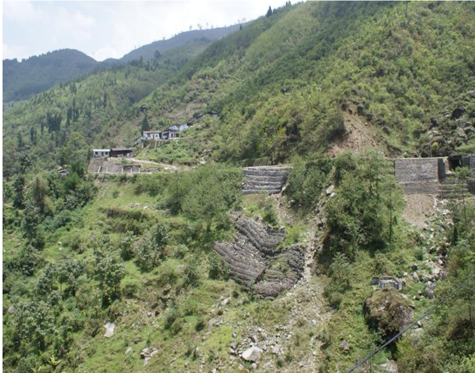
Figure 2. Bakthang falls landslide.
