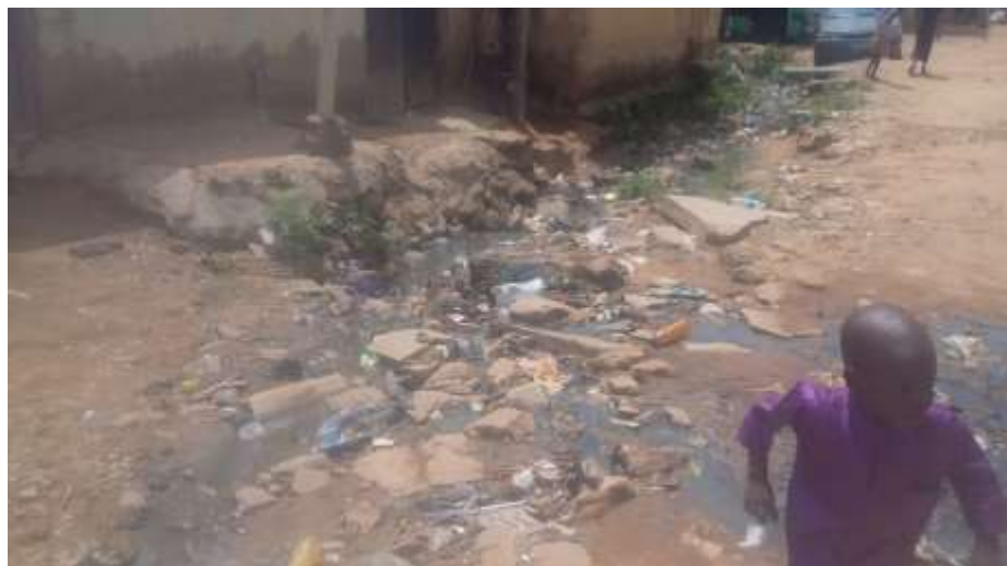
Plate 3. Open drainage. Source: Fieldwork, 2018.
