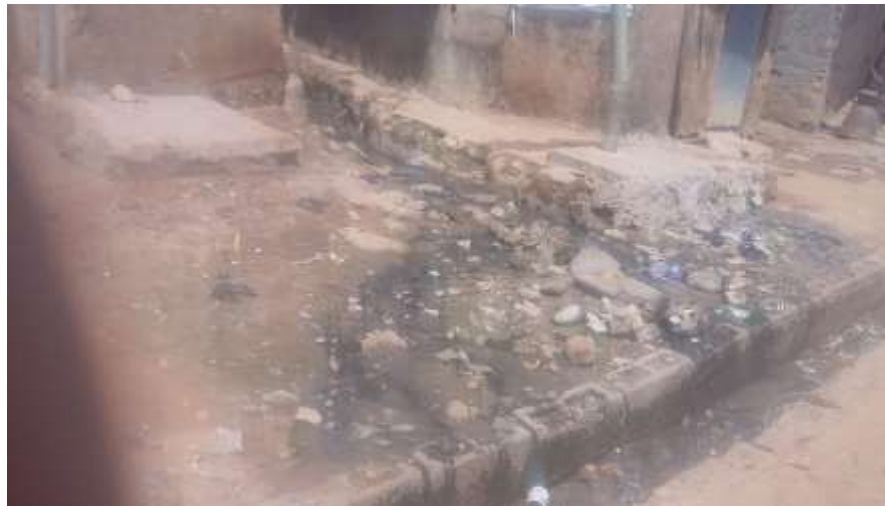
Plate 2. Open drainage. Source: Fieldwork, 2018.
