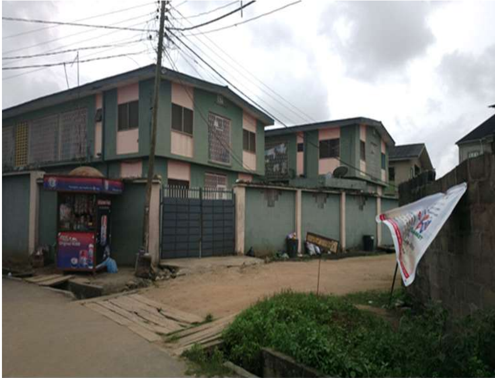
Figure 3. Picture showing the standard of structures and observed setback between structures in the private Estate.
