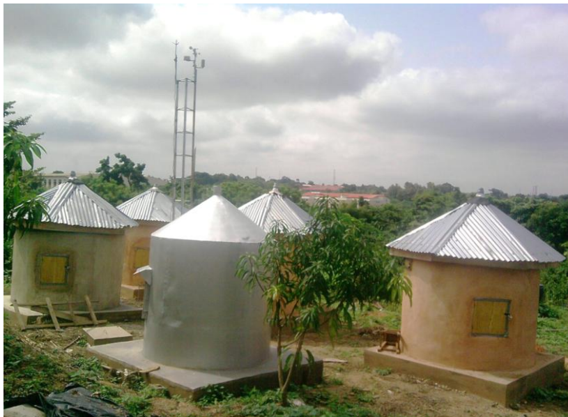
Figure 1. Picture of the completed experimental site showing the termite mound clay silo (front, right-most), reinforced concrete silo (front, left-most) and galvanized steel silo (front, center) with the adjacent weather station (back showing weather vane).
