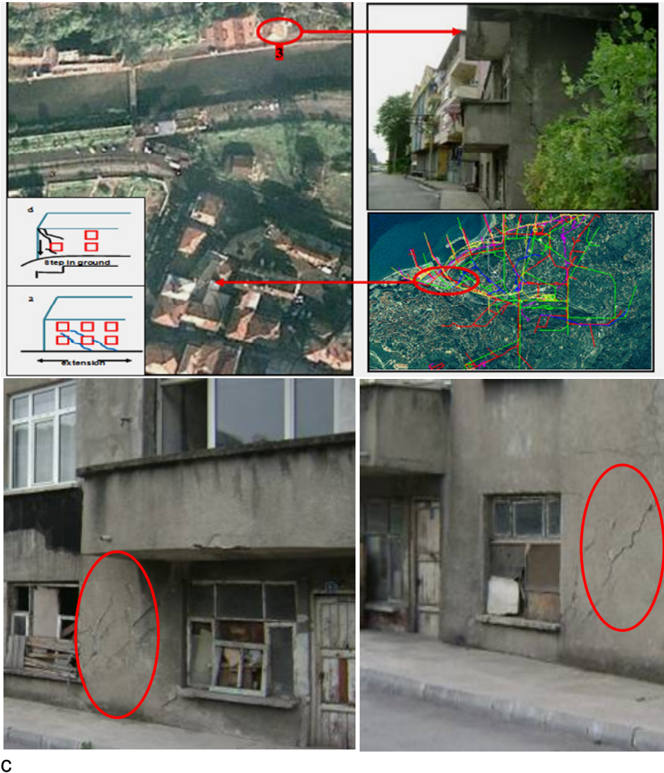
Figure 8a. Image and location of structural damage on building 1. (b) Image and location of structural damage on building 2. (c) Image and location of structural damage on building 3
